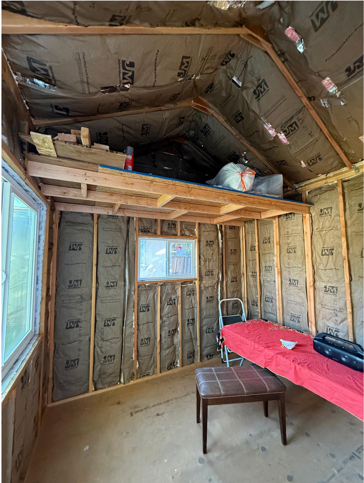
Figure 10: Interior Insulation Left Side
