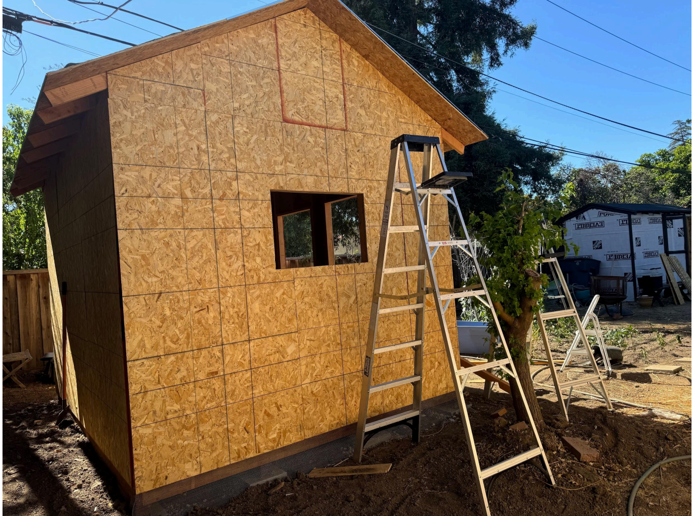
Figure 7: Side view of all plywood siding
