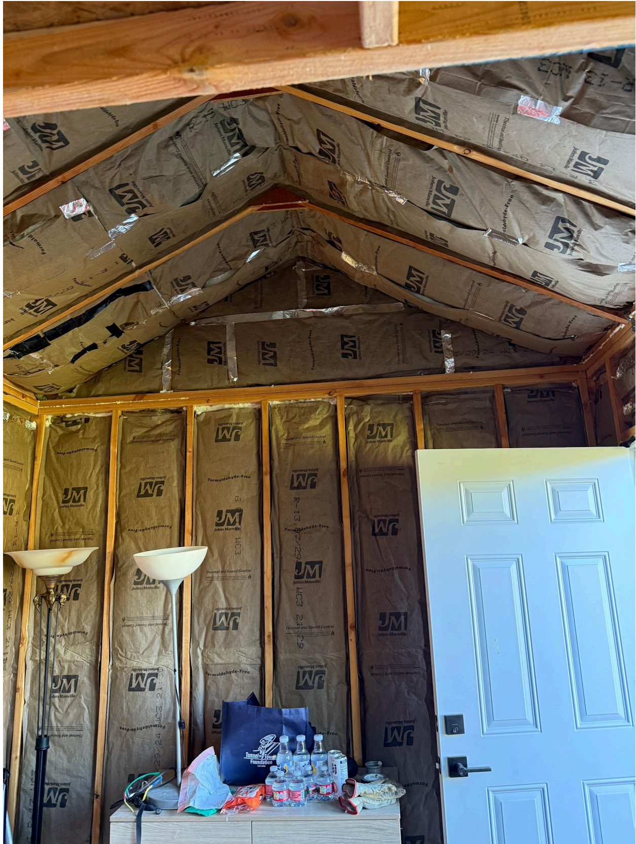
Figure 9: Interior Insuation Right side
