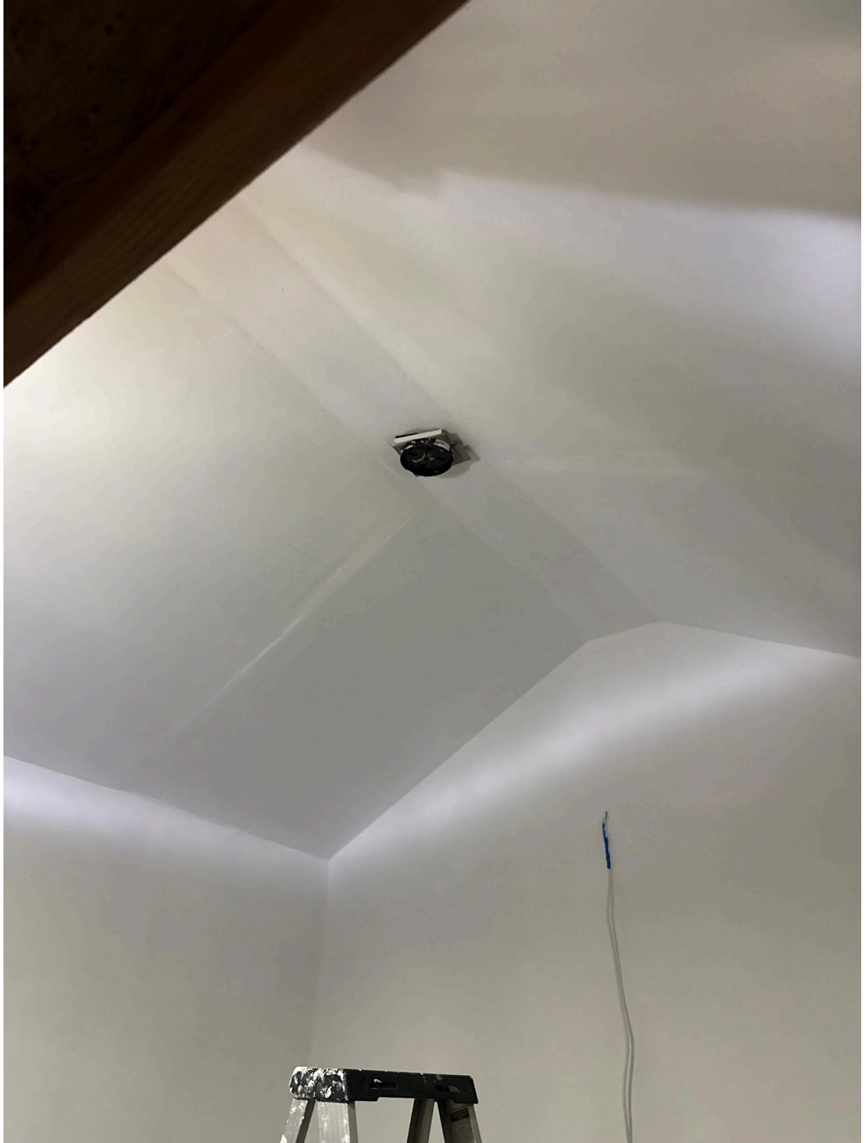
Figure 13: All sides painted, applying ceiling fan
