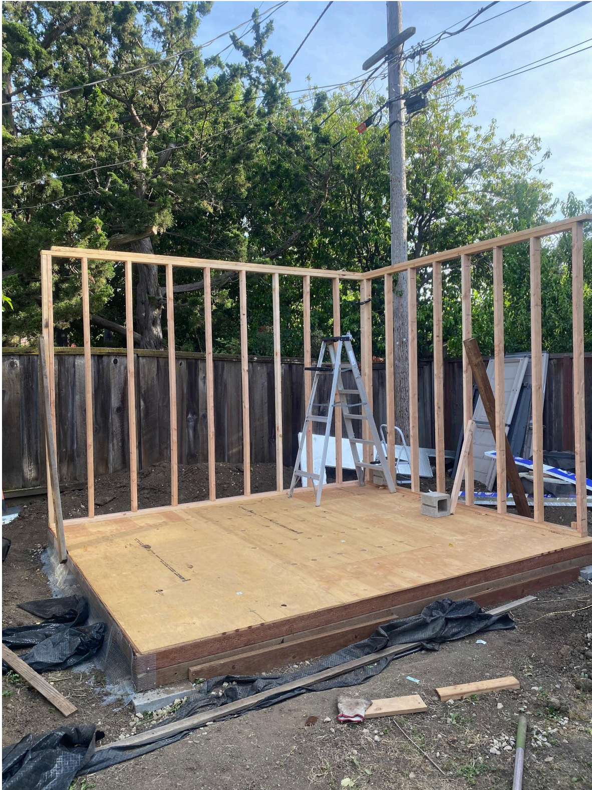
Figure 2: Installed Insulation under OSB board and wired/boarded edges for rodent protection. Added two of four frames
