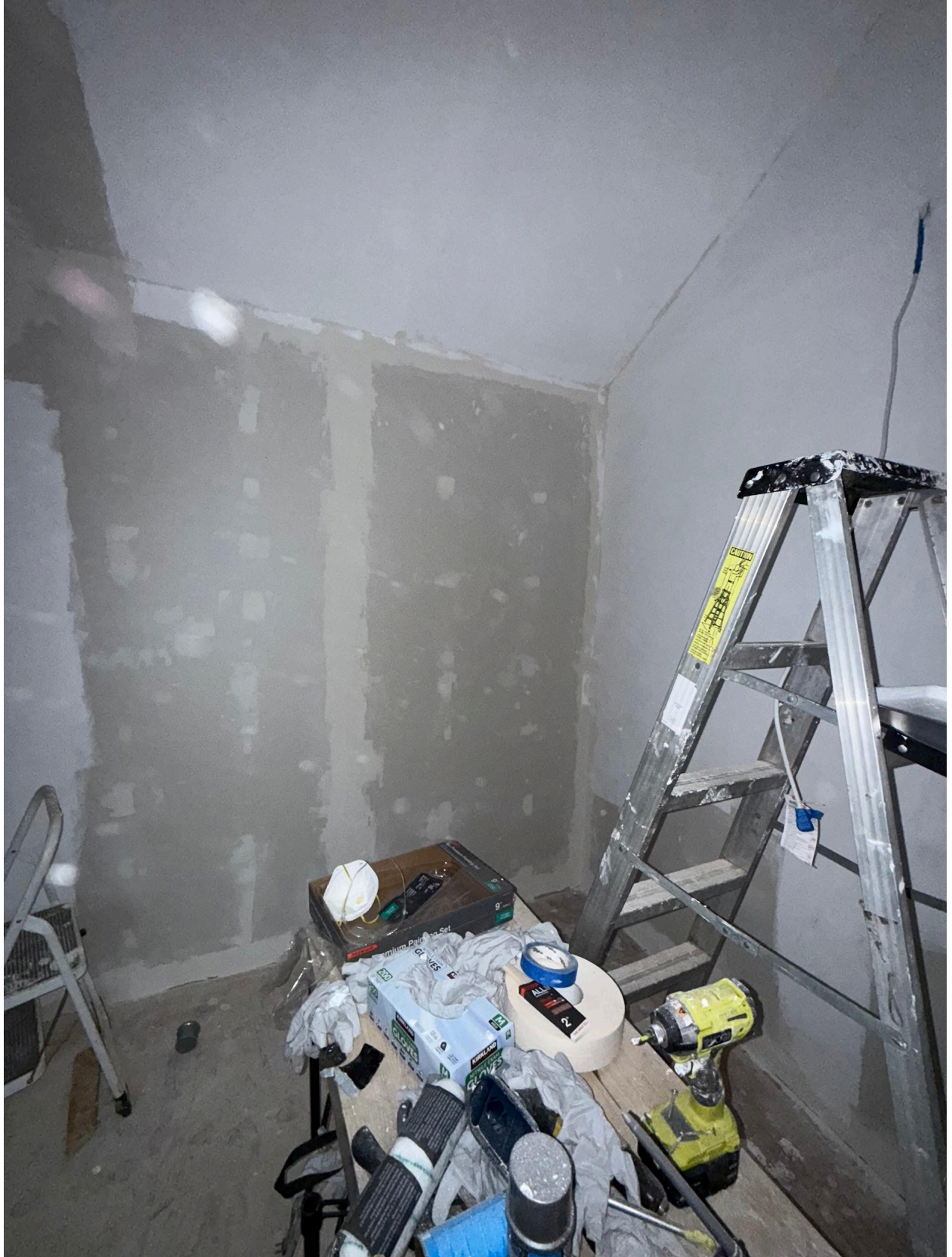
Figure 11: Drywall and plaster applied
