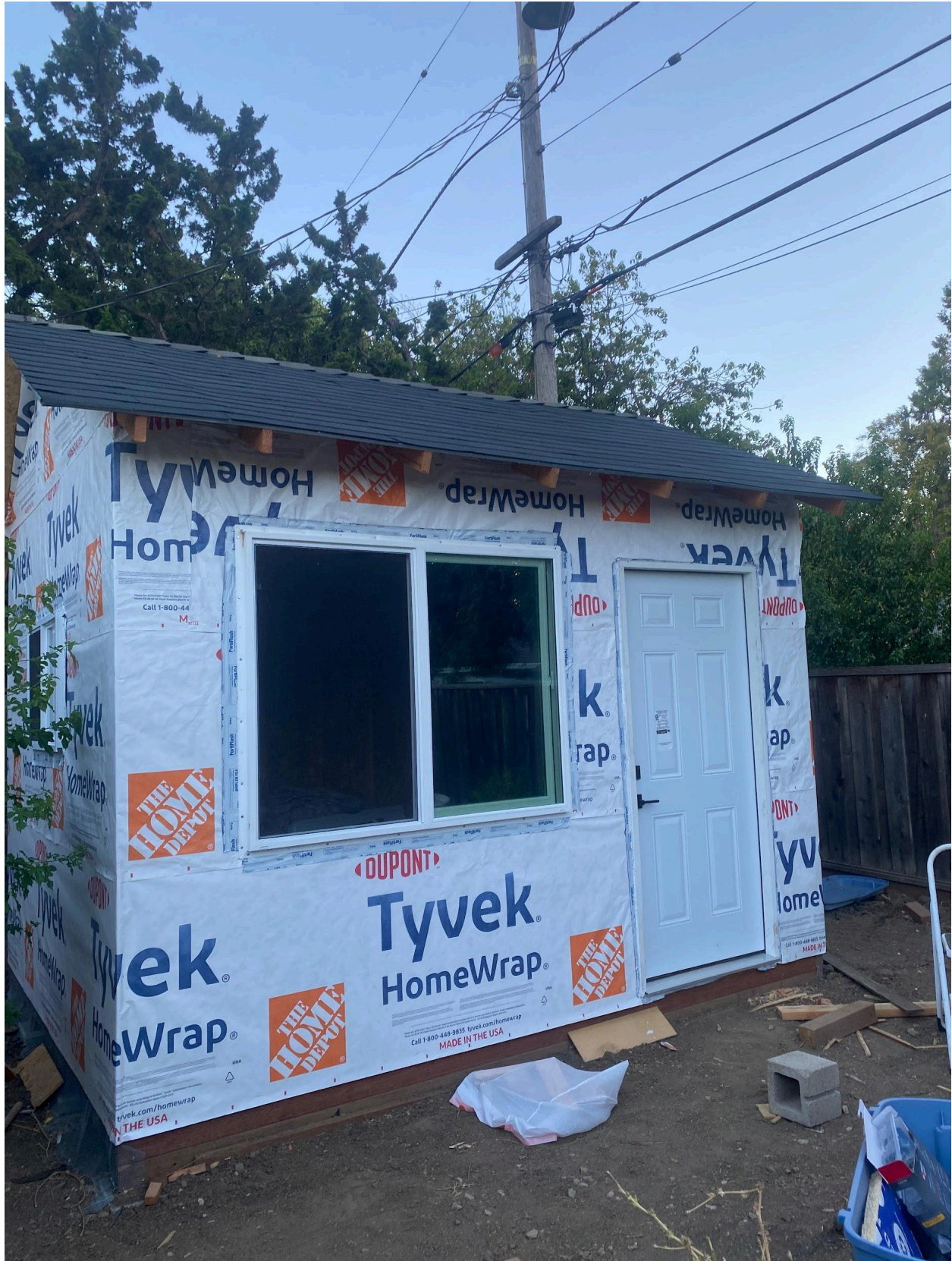
Figure 8: Installed all windows/doors with Tyvek weather wrap
