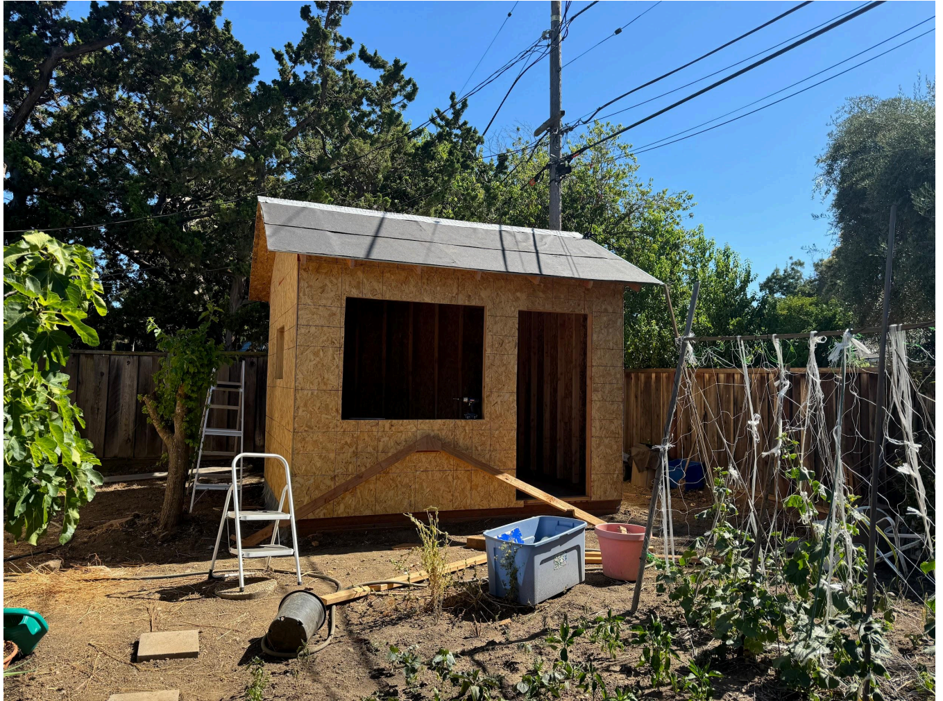
Figure 6: Installed Roofing Felt and prepped for shingles
