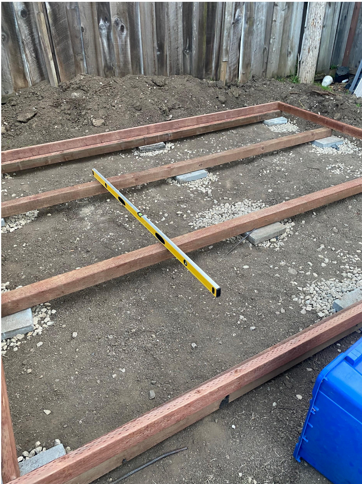
Figure 1.3: Continued Base, 4 cross beams, each supported by a 6 in gravel base and cement block
