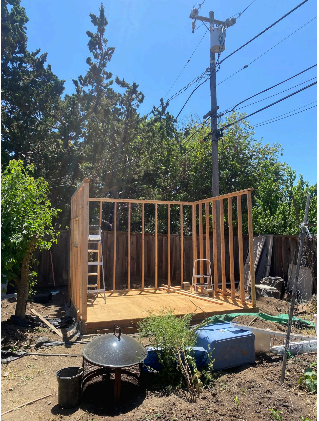
Figure 3: Installed 3rd Frame
