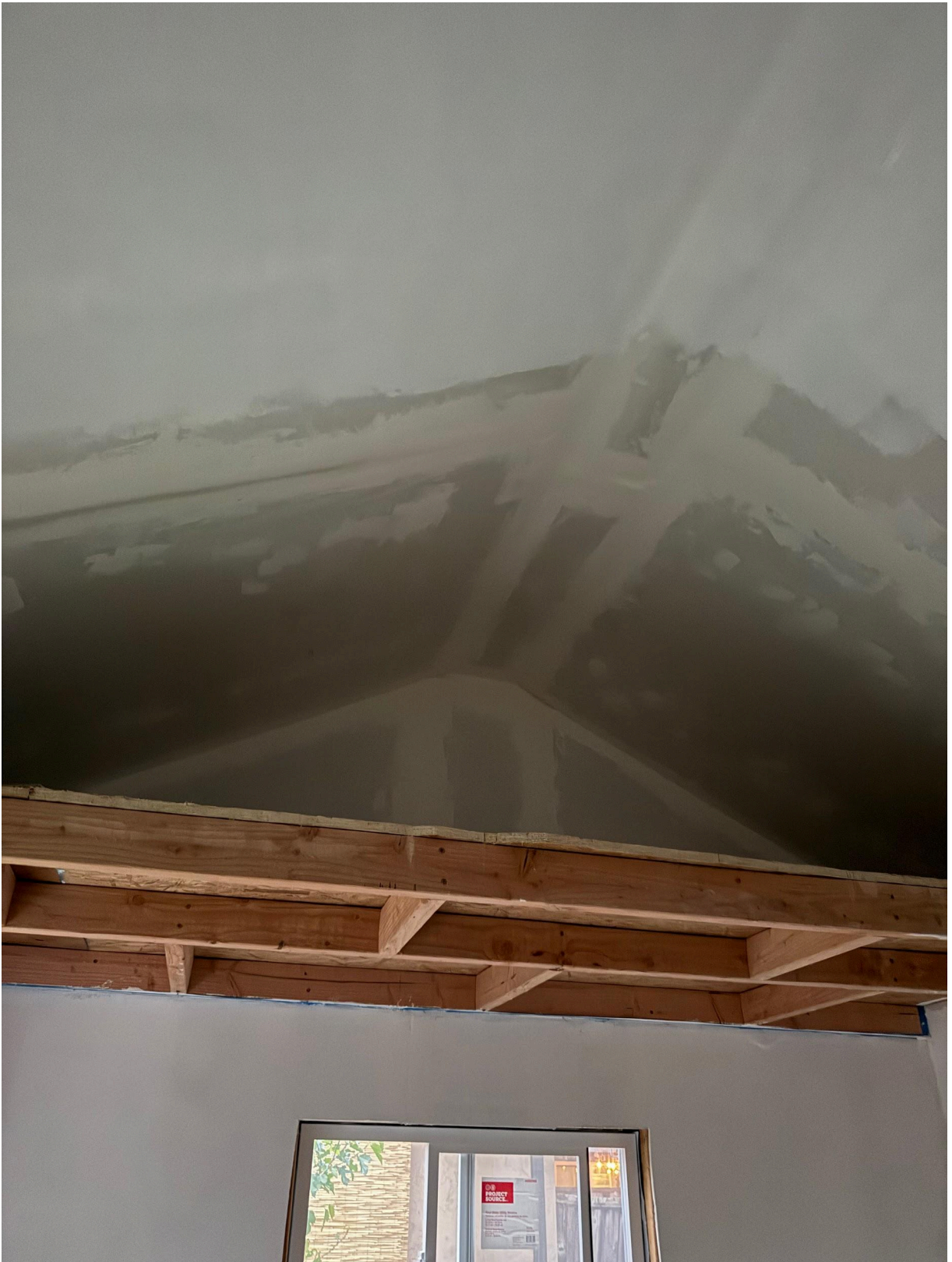
Figure 12.1: Drywall and plaster applied
